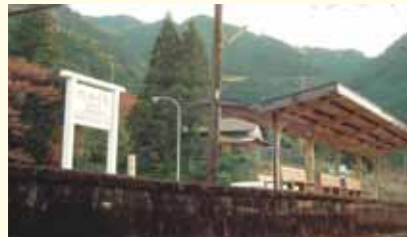
A platform shed and wooden bench
